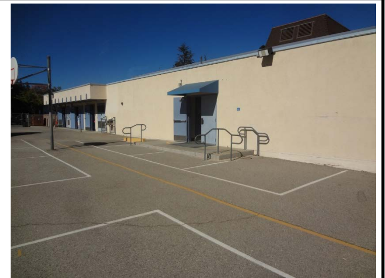
Photo -8 Back of MPR The backside of the MPR has accessibility issues as well as a lack of shading.
