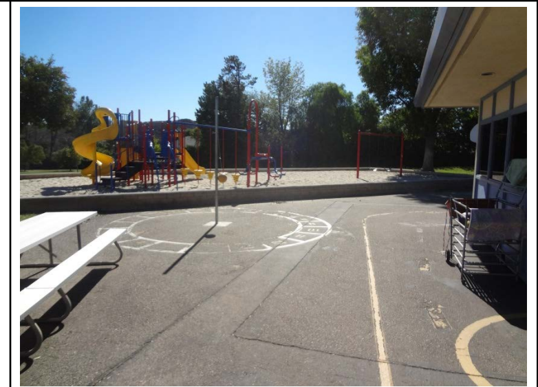
Photo -8 Curb Appeal – Kindergarten Play Area Kindergarten play area is efficiently laid out next to the kindergarten building.
