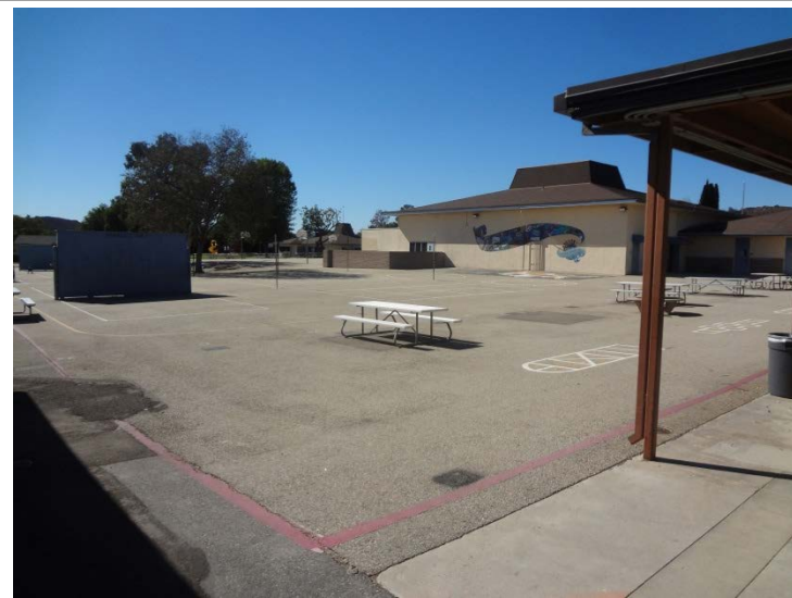
Photo -6 Lack of Shading The campus has large amounts of black top area with little shading from trees or buildings.
