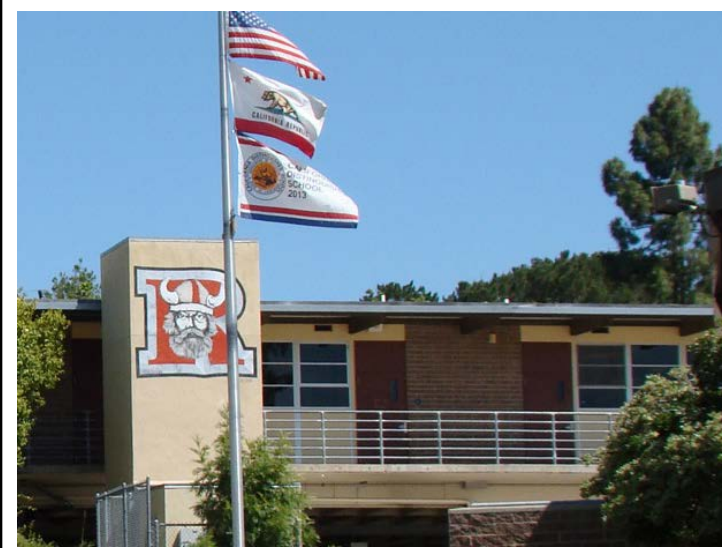
Photo -15 Elevator The elevator has not been certified through DSA.
