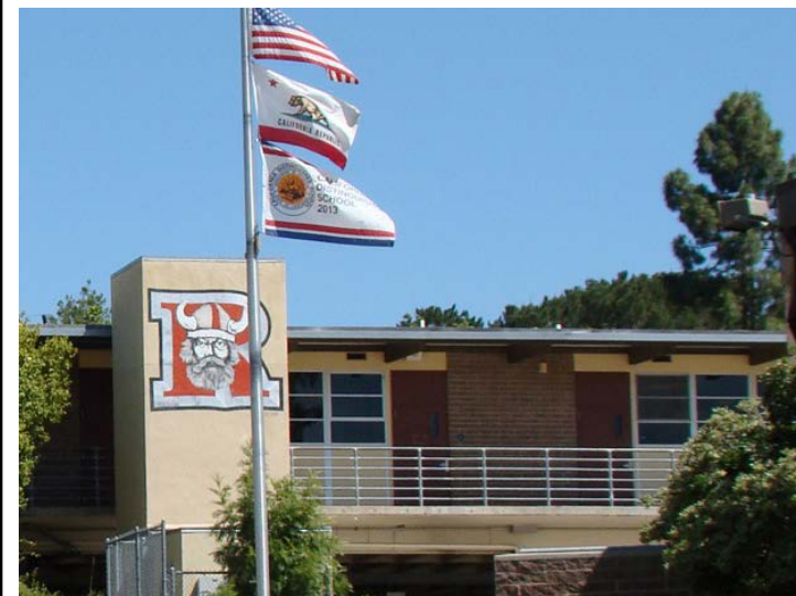
Photo -7 Curb Appeal – Elevated Classrooms The elevator with the school logo helps create symmetry for the elevated classroom buildings.
