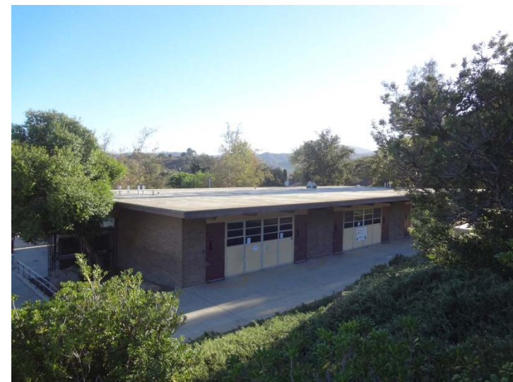
Photo -5 Curb Appeal – View of Classrooms Classroom buildings with split face CMU façade and are nestled into the hillside with mature foliage.
