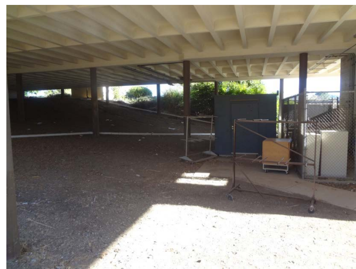
Photo -13 Fencing Beneath Classroom Building There is a need for fencing under the classroom buildings to increase security.
